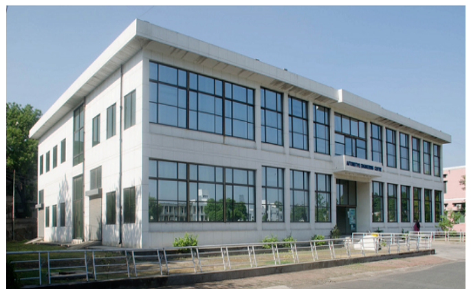
Fig. 1. Automotive Center, University of Engineering and
