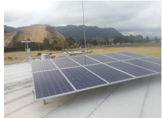
Fig. 4. Solar panel installation in Cajicá.
