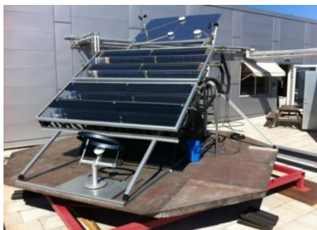
Fig. 3: Picture shows how the Thermal collectors were installed
