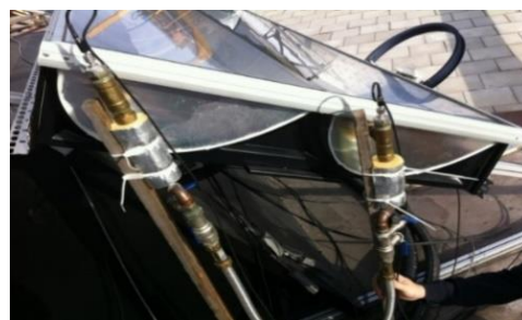
Fig. 5: Collector inlet side with Pt 100 sensors inside
