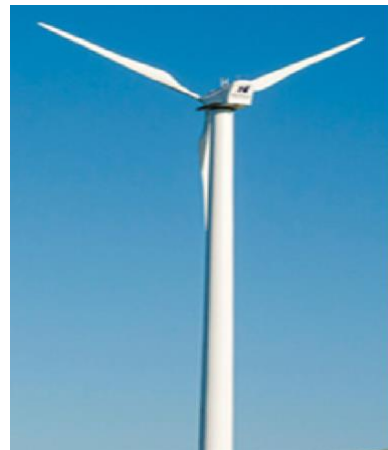
Fig. 1. WindPACT 1.5 MW Wind Turbine [35]
