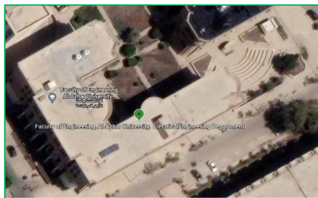
Fig. 14 Map of electrical engineering building in AL-Azhar university generated from Google Earth TM.
