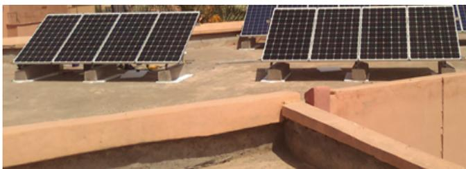
Fig. 1. The GCPV system installed at the Faculty of Science Semlalia Marrakech
