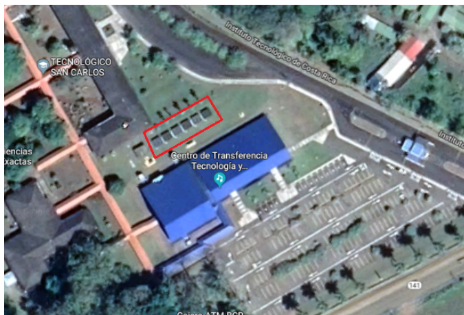
Fig. 5. Aerial photograph of TEC's photovoltaic station (identified in red) located in San Carlos. Source: Google Maps.
