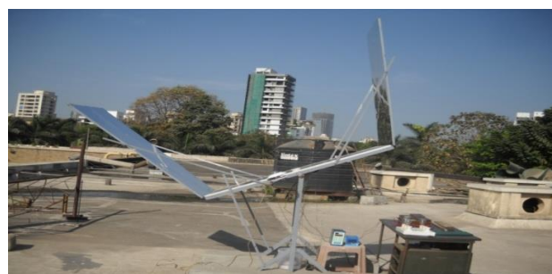
Fig. 1. Actual installation of flat reflectors to sides of PV module at N-S direction.
