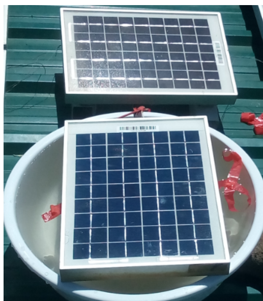
Fig. 9. Roof mounted air-cooled PV and water-cooled PV-TEG field setup
